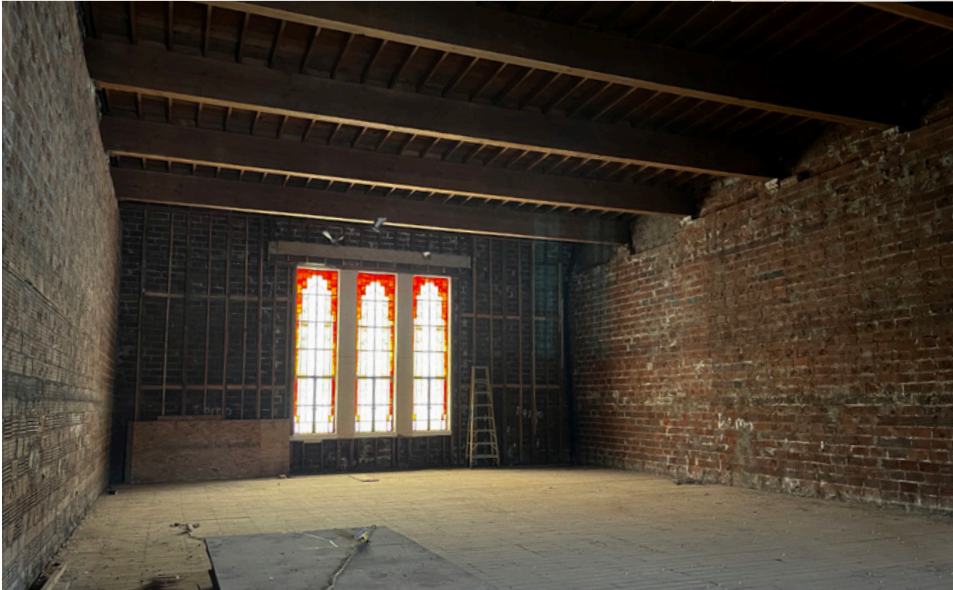
3RD Floor | Former Chapel
